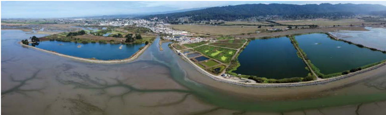
Arcata Wastewater Treatment Facility
