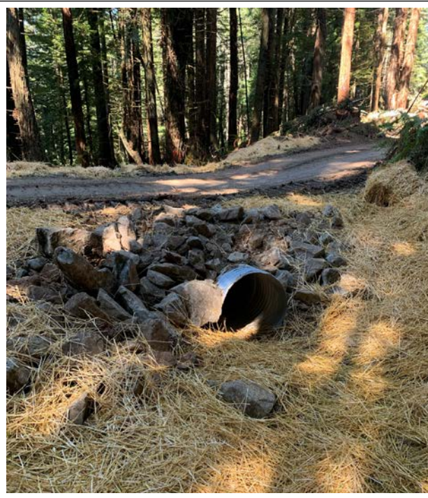
Timber Harvest 2022: New rocked road & new culvert installation (JCF Tract; Kline LaForge parcel)
