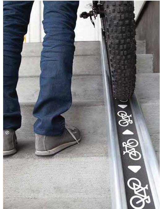
Photo 18: A bike channel by CycleSafe can be added to existing stairways, if the stairs are not too steep or narrow
