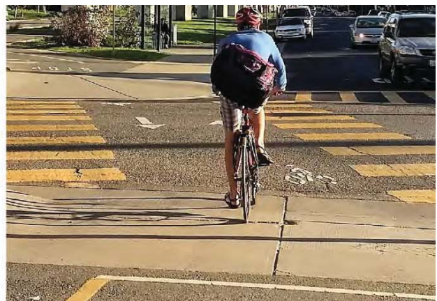
Figure 29: A high-visibility crosswalk with bike markings explicitly allows bicycles and alerts drivers to additional users.
